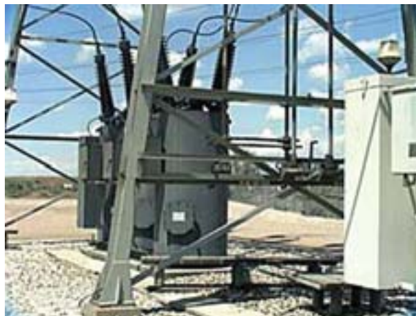
Oil circuit breaker
